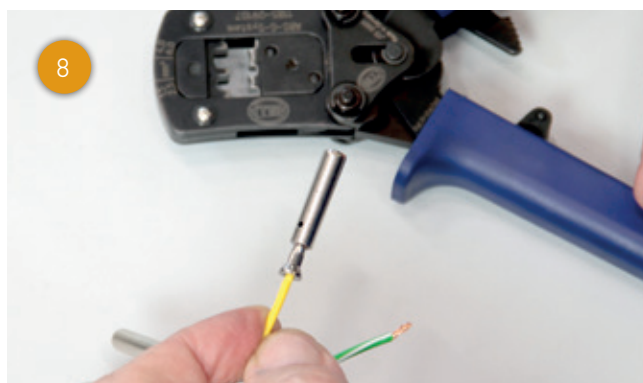
8 Repeat this procedure for all the vehicle cables required.
